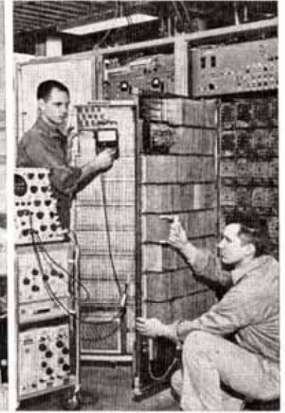
PRODUCT SERVICE Technicians at the BMEWS site, R. Braun, (kneeling) and H. Brewington (standing), check out the synchronizer, which controls operation of the complex transmitter-receiver.
