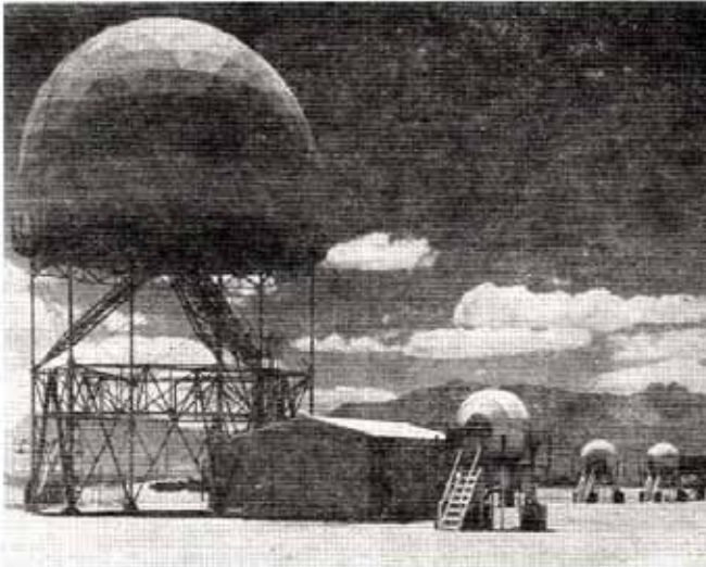
HIPAR RADAR—U.S. Army's Improved NIKE-HERCULES System at White Sands Missile Range, New Mexico, showing General Electric-built high power acquisition radar (HIPAR) housed in large radome and tracking radars built by Western Electric Company, prime contractor for the NIKE-HERCULES System. These advanced radars played a key role in last Friday's destruction of a Hercules missile by another Hercules missile.
