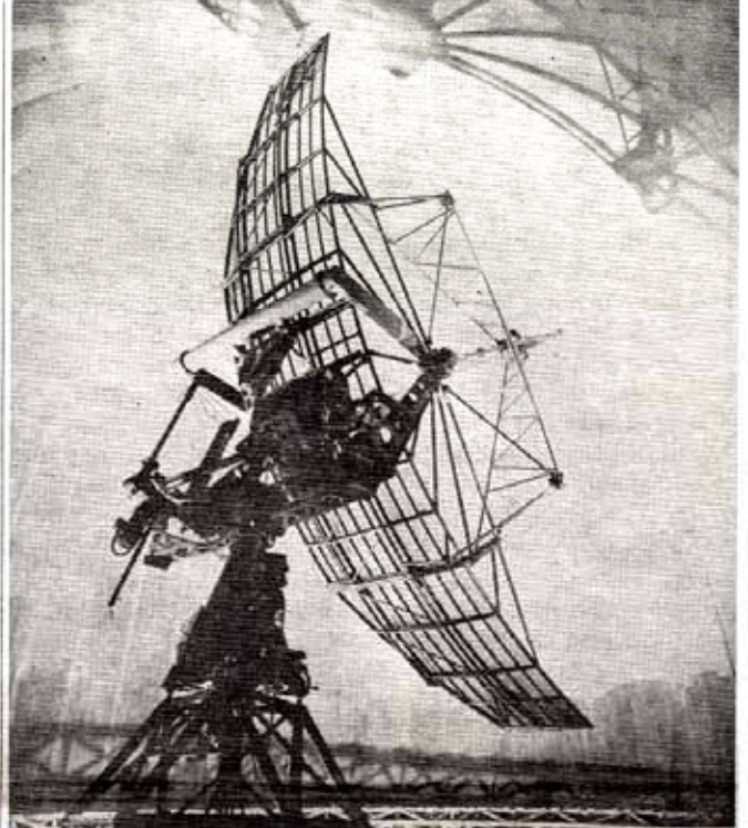
SYRACUSE-BUILT RADARS — Heavy Military Electronics Department here has been awarded a $2½ million contract for anti-jamming modification kits to be installed on these AN/FPS-6 Height Finding Radars. The AN/FPS-6 radars provide USAF installations throughout the Free World with long range, accurate height information on air targets several hundred miles away.
