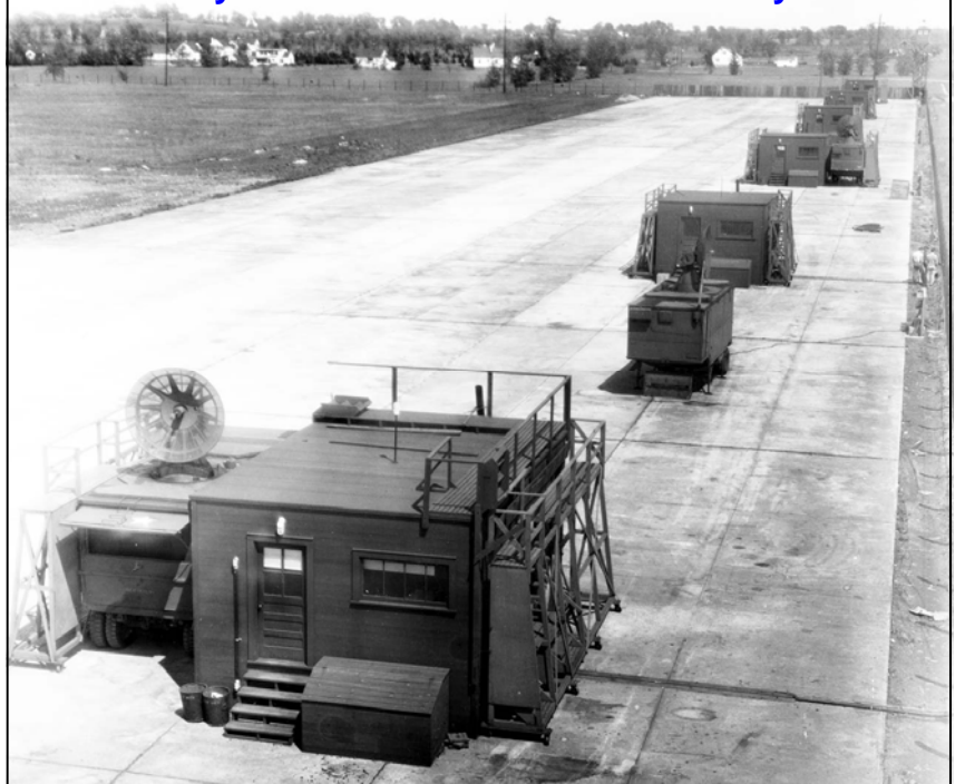
SCR-584 Systems Test on Wolf Street in May 1944
