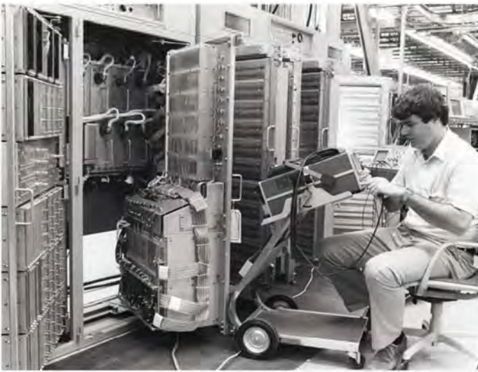
November 6, 1984 - Cabinets for the Over-The-Horizon (OTH) radar system undergoing checkout in the Farrell Road Building 2 cabinet test area.
