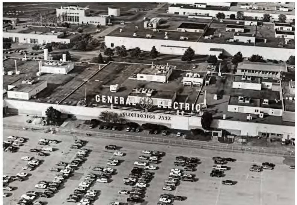
September 30, 1990 - Aerial view of General Electric plant in Liverpool, NY. Buildings on the right hand side (front to back) are Building 7, Building 6 and Building 5. Building 10, the Power House, is at the upper left hand corner of the photo.
