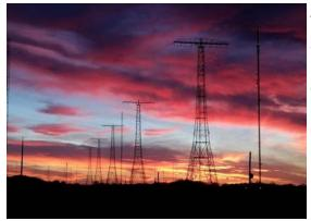
To obtain efficient transmission of the radio signal generated by the alternator's low frequency, a very large **Antenna** which consists of six 400+ foot towers with 150 foot crossarms supporting a multi-wire antenna is used. (This photo looks a bit like some of the sunset photos of GE's OTH Radar antennas - different frequency range, though.)
